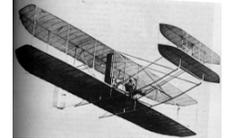
The only propellers they had ever seen were on boats, and they are always at the back. The same is true for the rudder. They are always at the back. However, the rudder on a boat is pushing against water, a much more dense fluid than air. So the Wright brothers put their rudder out on the end of a boom in order to benefit from the Lever Principle. That is another good Cause & Effect example that you can use.
